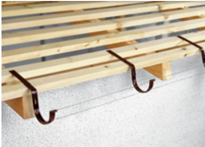
Installation of top rafter steel brackets
